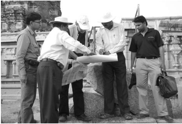
Figure 2. Conservation specialist John Hurd (center) reviews the drawings with the local Jindal Steel engineer T.S. Gowda ( left ) and the Kannada state archaeological team to determine the best manner in which to proceed with the embankment stabilization of Chandramauleswar Temple ( rear ), in India. Seeking in-country support from major donors is key to Global Heritage Fund success
