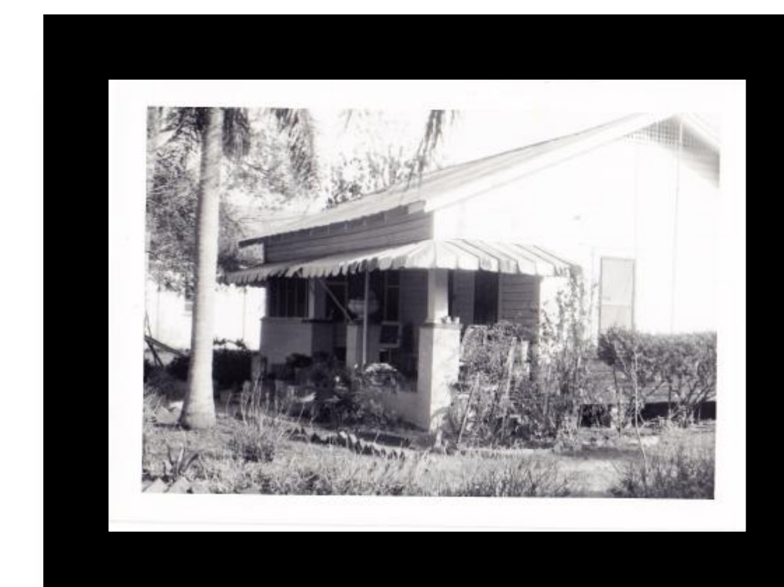
Figure 7. Spring Hill home torn down by interstate and urban renewal. Photo courtesy: Mr. Willie Streeter.
